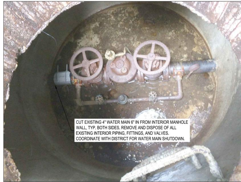
CUT EXISTING 4" WATER MAIN 6" IN FROM INTERIOR MANHOLE WALL, TYP. BOTH SIDES. REMOVE AND DISPOSE OF ALL EXISTING INTERIOR PIPING, FITTINGS, AND VALVES. COORDINATE WITH DISTRICT FOR WATER MAIN SHUTDOWN.
