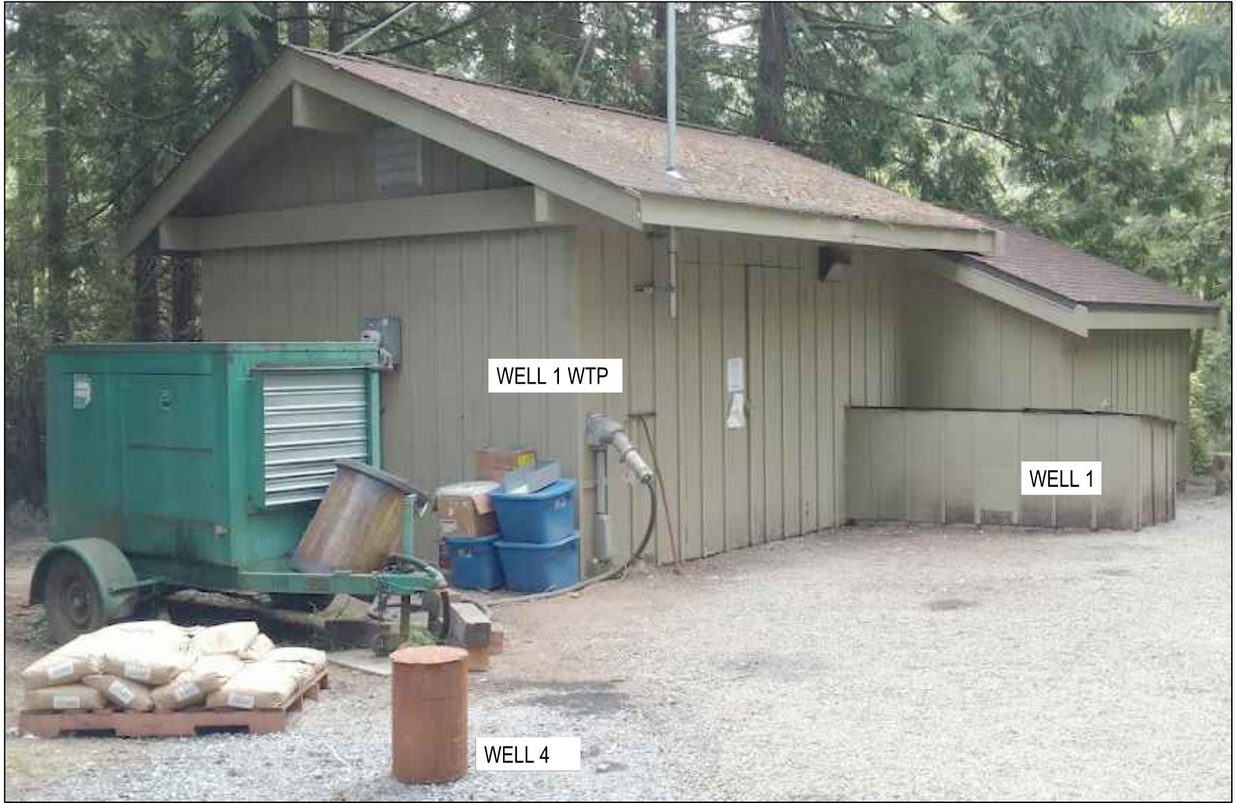
WELL 1 WTP AND WELL 4
