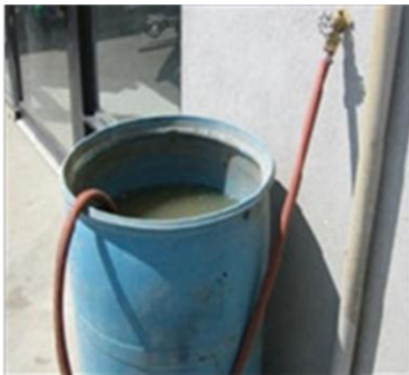
Submerged hoses can act as a conduit for contaminants under backflow conditions.
