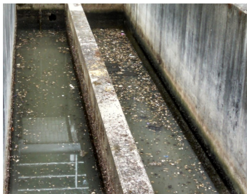
The old, larger screens allowed large quantities of refuse to enter the plant.
