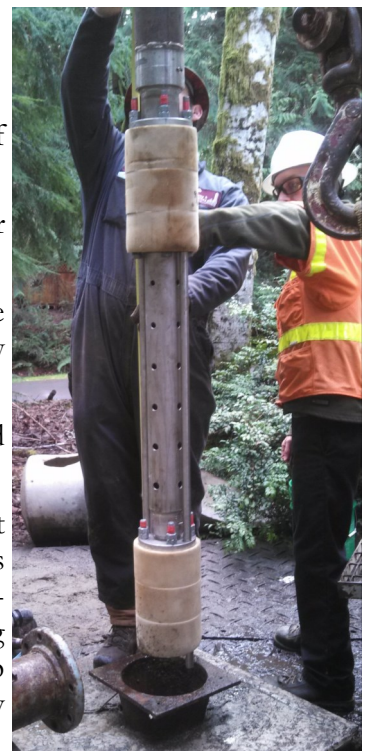
De-sanding tool being inserted into Well 1.
