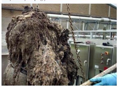
Non-flushable items cannot breakdown & buildup in equipment over time, requiring removal by operators and replacing equipment
