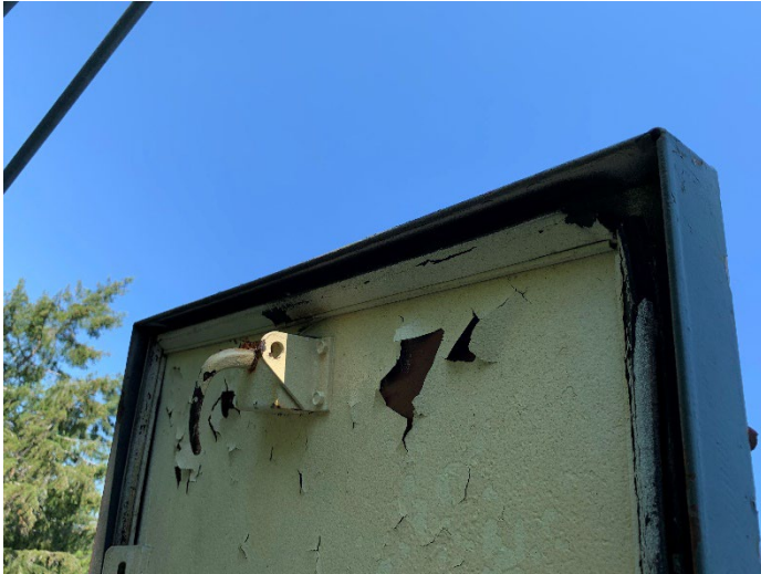
Underside of hatch with intact perimeter gasket
