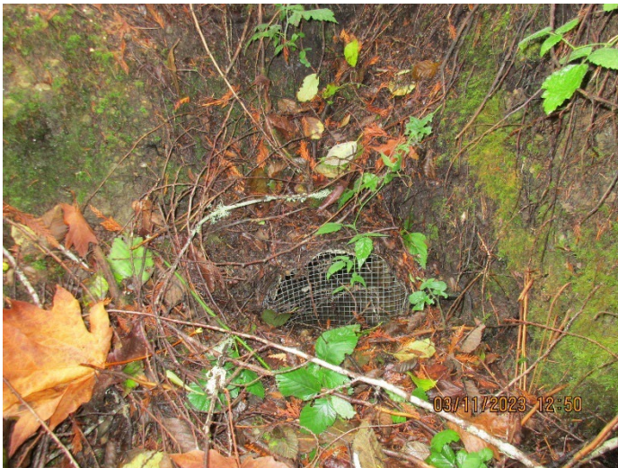
Reservoir overflow outlet with secure screen
