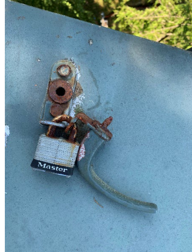
Latch will be replaced, and underside of hatch repainted in spring of 2024
