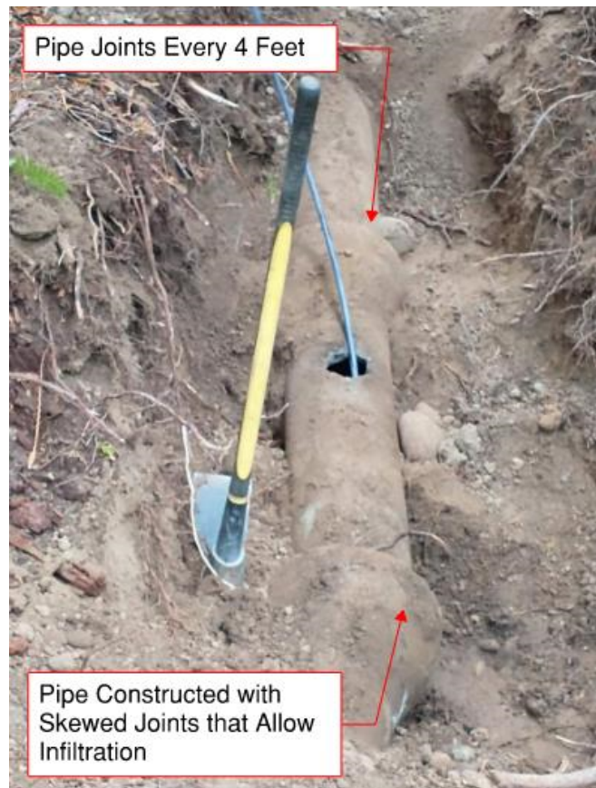
Figure 2-2: Existing HPWSD Pipe
